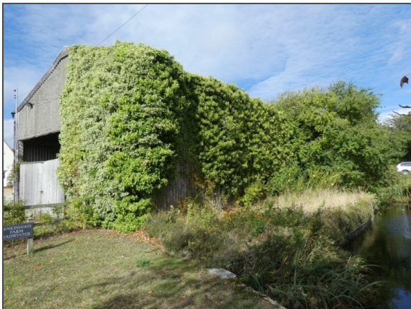
Overgrown roadside elevation
