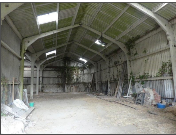
Interior, main barn
